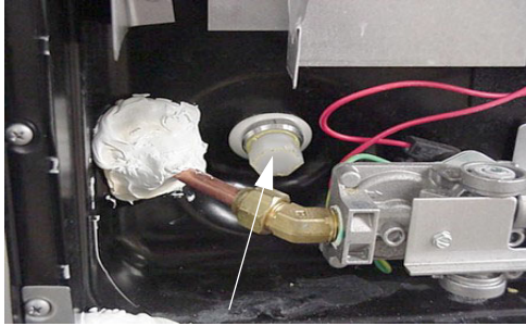
Water Heater Drain Plug (Remove with socket)
